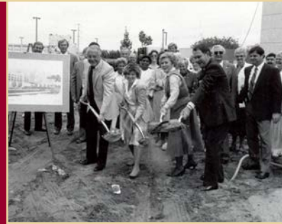
Construction begins on the North Patient Tower
