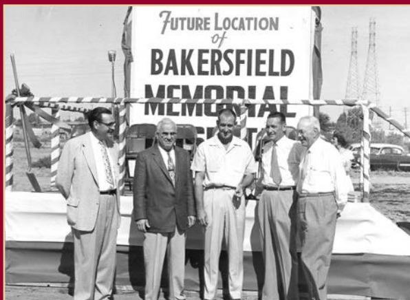
Construction begins on Bakersfield Memorial Hospital on 34th Street.
